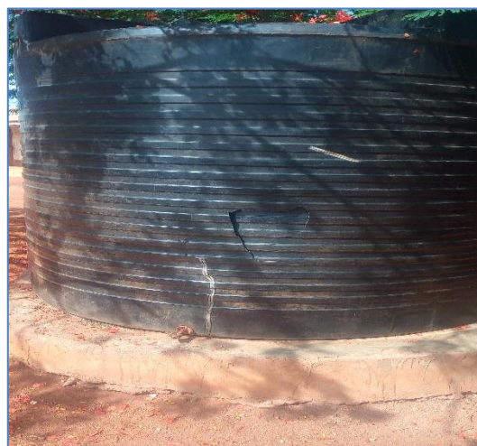
Storage tank at Msharinyi Primary school alleged to have been speared by a member of the local community after realizing it had no water
