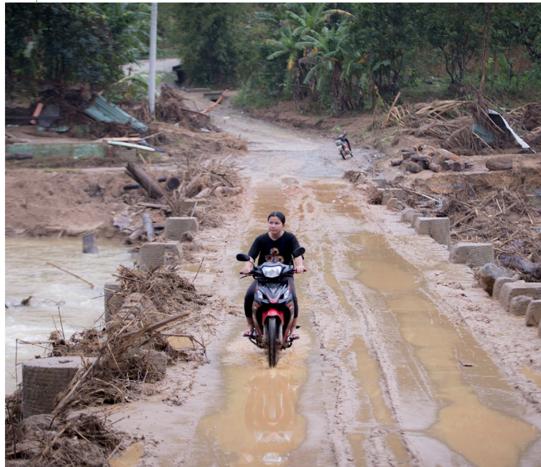
A woman rides a motorbike over a damaged bridge that leads to landslide-prone areas in Nam Tra My district, Quang Nam province, Vietnam.
